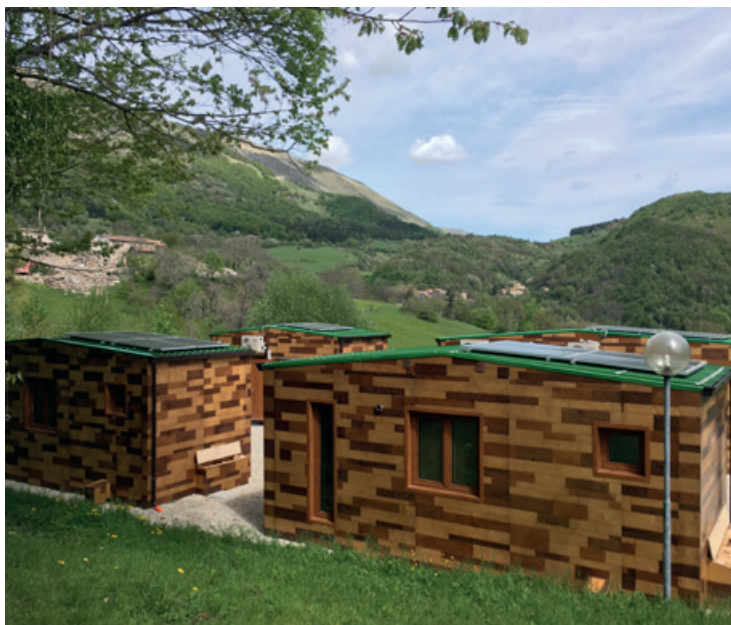
Temporary hiking shelter of Colle di Montegallo (ph PNMS)
